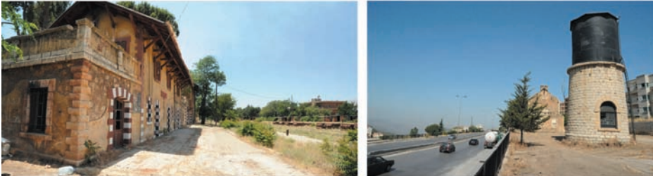
Photos 2-3 (top) and 4-5 (bottom): 2 (Abandoned railway facilities at Dahr El Baïdar Pass), 3 (Three parallel transportation axes near Jbail – Byblos-), 4 (Disused railway station at Rayak – Bekaa-) and 5 (Bhamdoun – Lebanon Mountains-: Damascus highway and former railway station) (Photos X. Bernier, June 2010)
